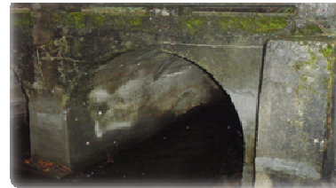
(Bowen Island Project after repair)
